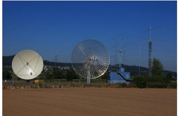
The antenna farm at HB9Q enables them to have great EME activity. It consists of a 15 m mesh dish for 144 and 432 MHz, a 10 m solid dish for 1296, 23xx, 3400, 5760, and 10xxx MHz, 8x19xxx M2 Yagis for 144 MHz, and 1x2.5wl M2 Yagi for 50 MHz, on top of the HF beam, 24 m above ground. (Photo by HB9CRQ)
